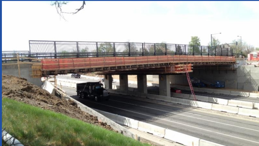
New, nearly complete Knox Court bridge
